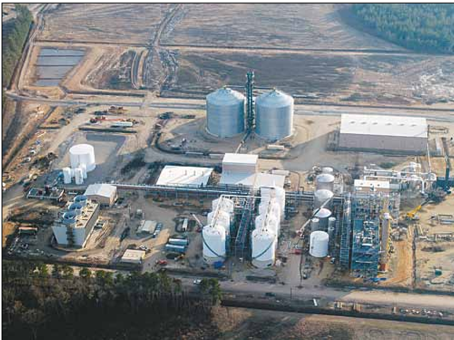
The former Clean Burn Fuels ethanol plant when it neared completion. It operated for only a few months.
