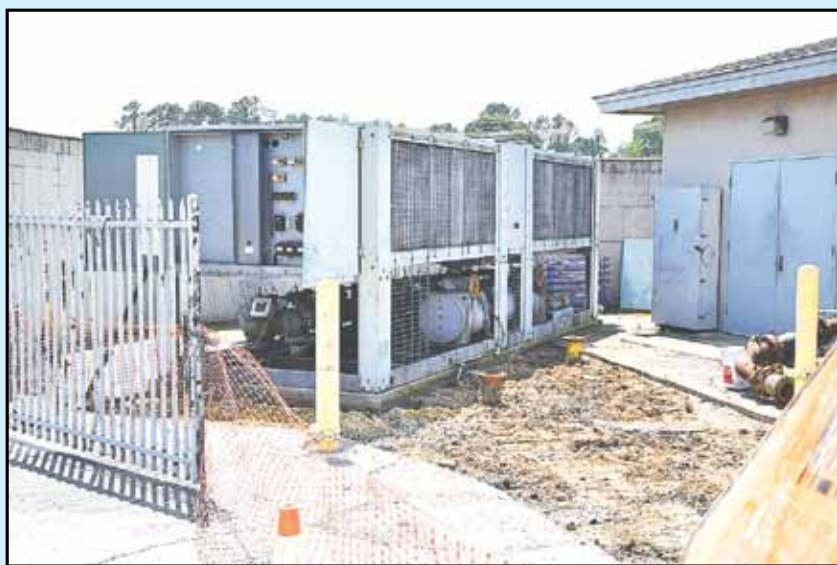
Fans suffice, but just barely, in the office at Rockfish Hoke Elementary School. At left, the old chiller is being removed and a new one installed. (Ken MacDonald photos)
