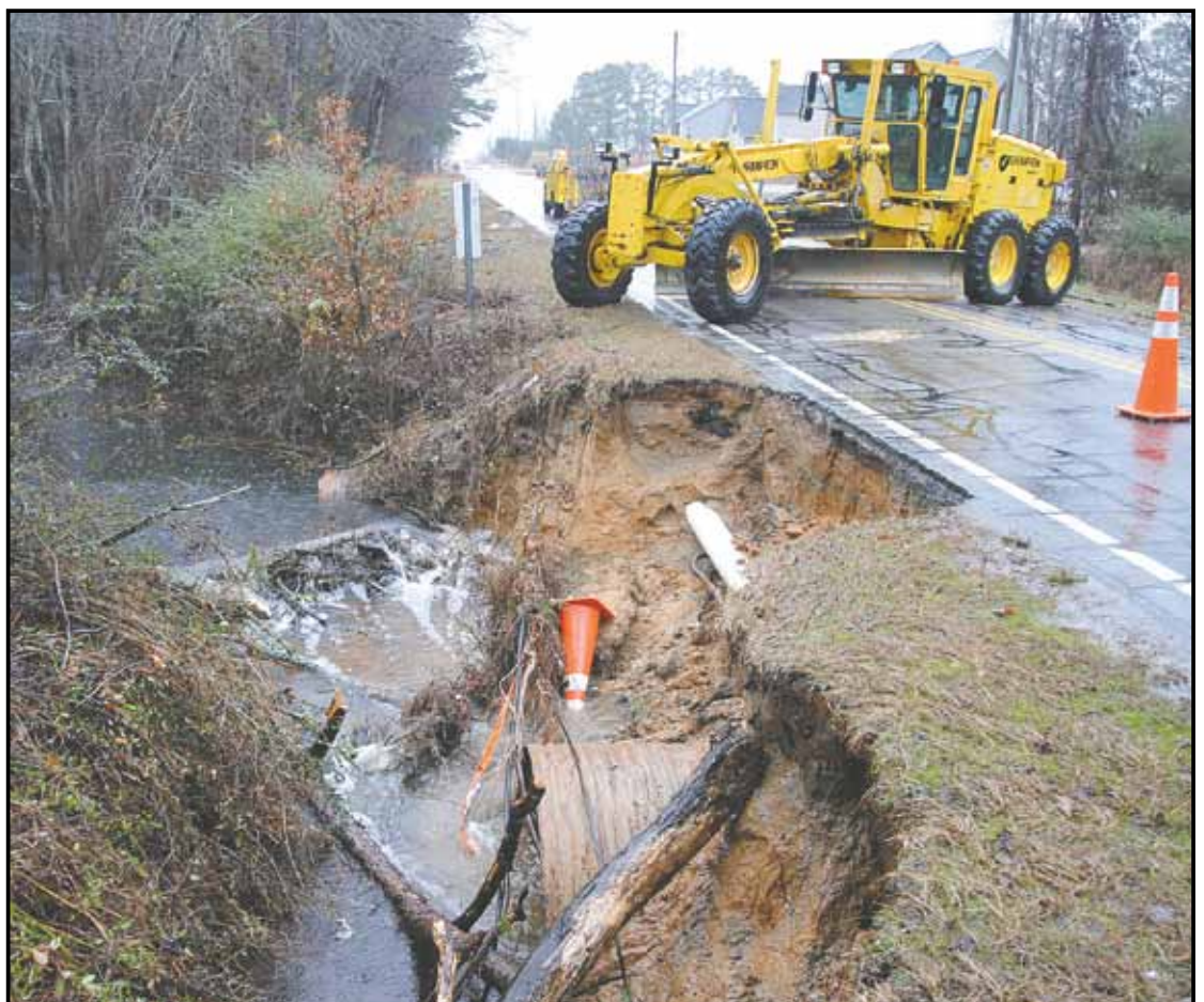
DOT crews blocked Lindsay Road after it was washed out by flooding water Friday. The road remains closed between Stoney Point and Adcox roads. (Ken MacDonald photo)
