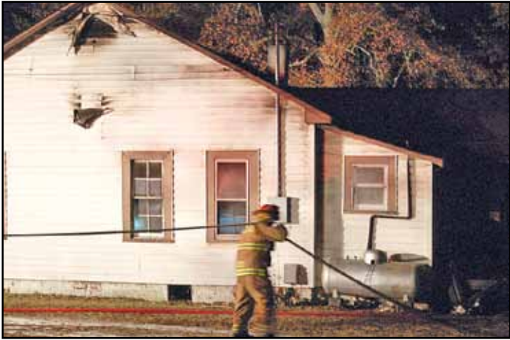
An explosion at this house was likely a backdraft.
