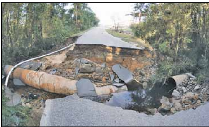
Steele Road, the only entrance to the transfer station.
